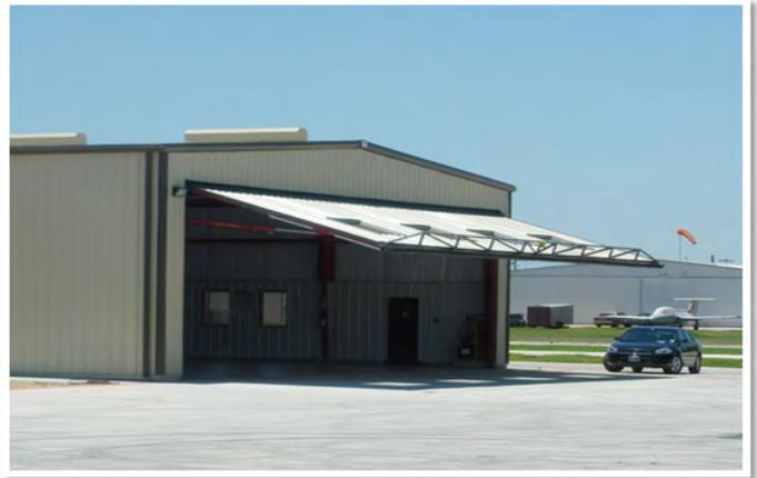
A Schweiss hydraulic door provides shade in front of the hangar when in the open position.
